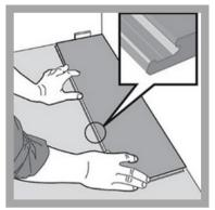
1) First plank, first row. Leave a 1/4" gap against all walls and position the plank tongue-side against the wall.
